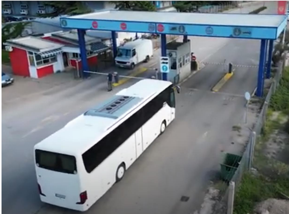
Figure 13- Port Security gate in the port of Bar
