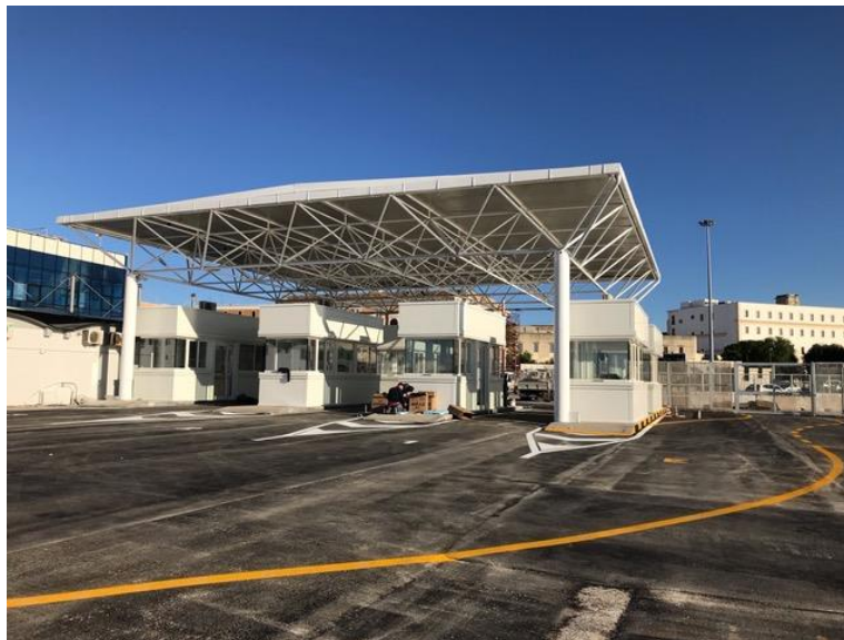
Figure 4- Vehicular and pedestrian gates at the San Vito port facility (AC1 gate)
